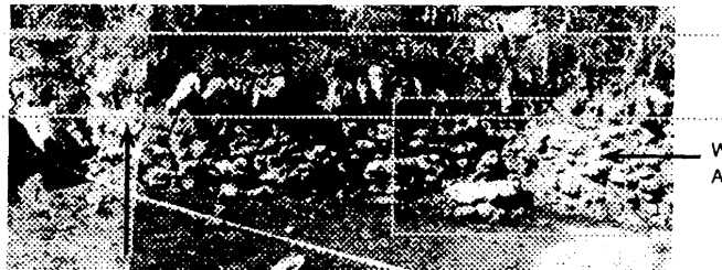
18 INVASIVE AND OVERGROWN CANE COMPROMISING STONE CAP. WALL IMPACTED BY ROCK SLIDES.
