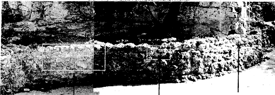
29 WALL CRACKED. STONE CAP MISSING OR DETERIORATING. LIMESTONE WALL DETERIORATING.
