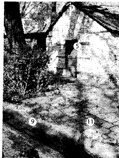
C4- Southeast corner
