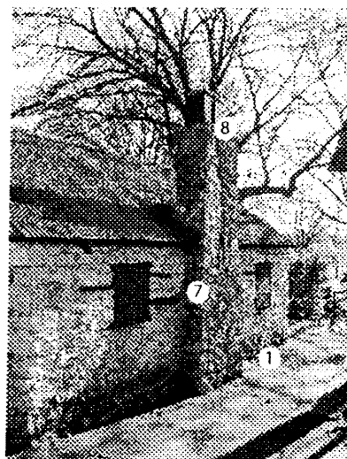
C11- West facade
