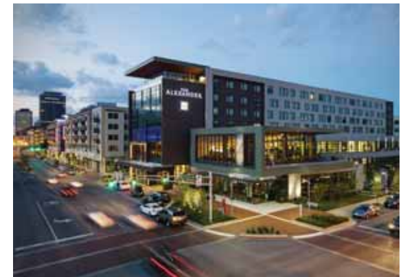
The Cityway development in downtown Indianapolis includes a world-class business hotel, high-end apartments, restaurants, retail shops and other community amenities.
