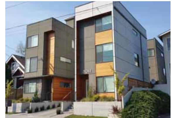
Stacked flats in Seattle, Washington integrate four well-designed residences into a standard single-family parcel.
